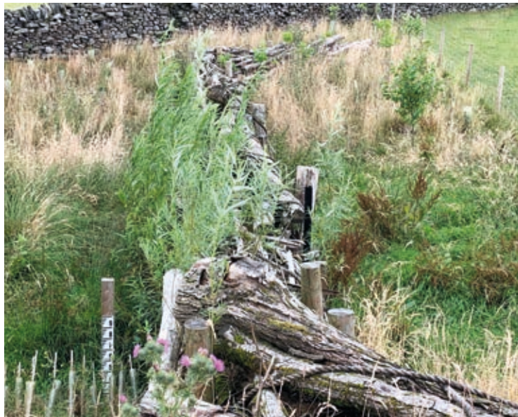
Leaky barrier at New Mills © Environment Agency
