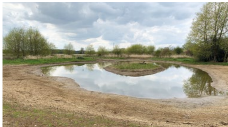
NFM storage pond in Leicestershire © Environment Agency
