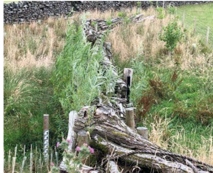
Leaky barrier at New Mills © Environment Agency
