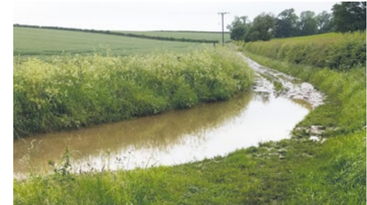
Slope erosion © Peter Haynes
