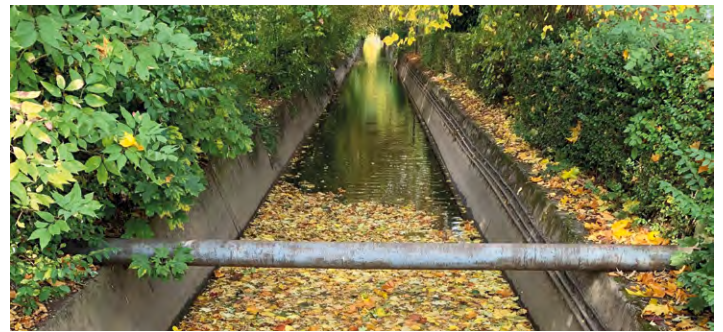
Engineered channel in Long Eaton © Mark Hamblin 2020VISION
