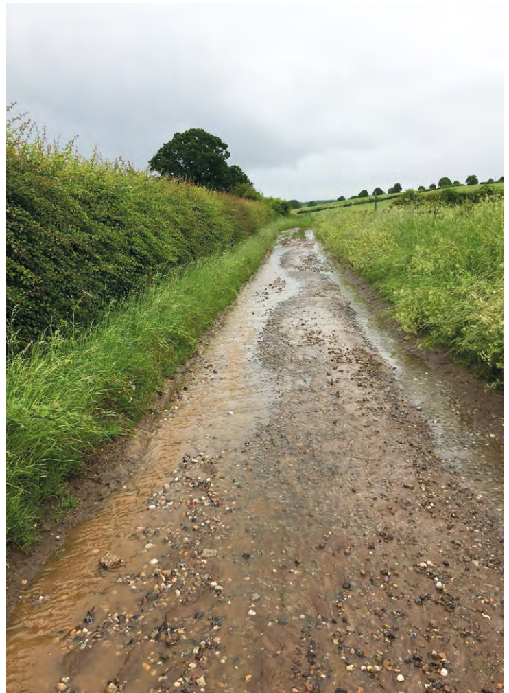
Pathway erosion © Peter Haynes
