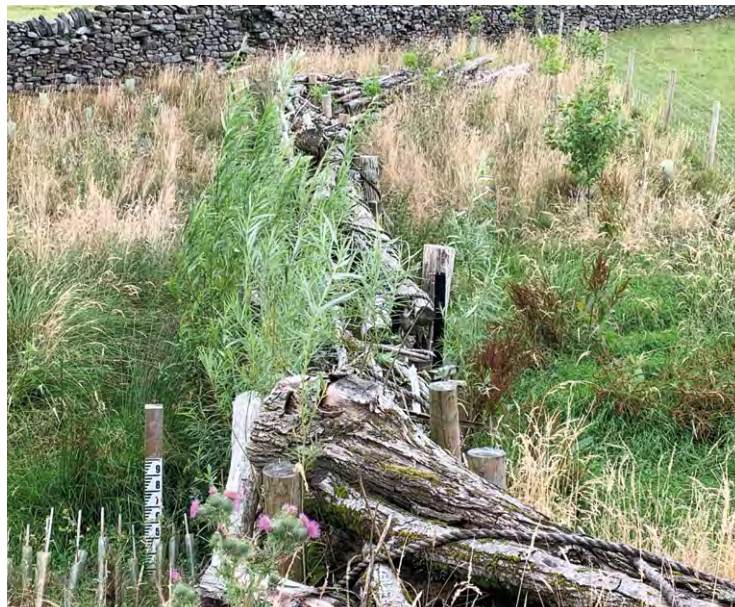
Leaky barrier at New Mills © Environment Agency
