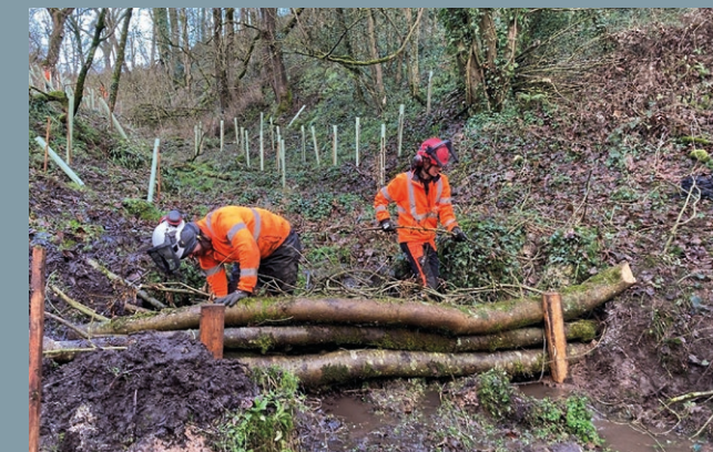
Leaky dam installation in the Derwent River Catchment. Photo: © Mark Young
